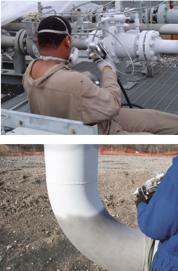
Figure 10: TSA are capable of being applied on different shapes and sizes of equipment with very good adhesion and reliability (“Copyright Sulzer Technical Review, Sulzer Management Ltd, Winterthur, Switzerland”. Used with permission)
